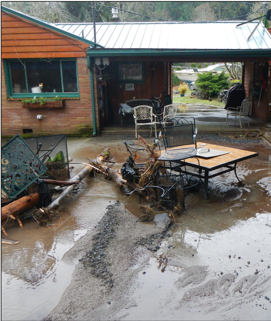
2014 lower Big Quilcene flood damage. Photo by Pat McCullough
